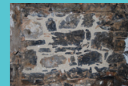
Prefugiranje zidov. Vir: Corradi in sod., 2006
